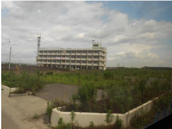
Elementary school that survived the tsunami
