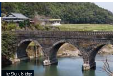
The Stone Bridge
